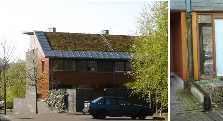
*Fig. 19. Left: Green roof with zinc edges. Right: Visibility of stormwater and zinc 'down-pipe'.*
